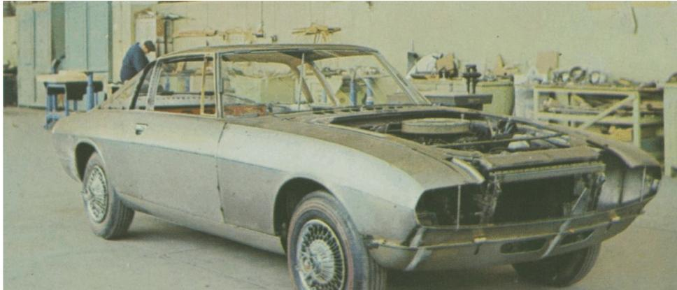
*This image, from the 1965 **Automobile Quarterly** article on the Scott Bailey Mustang, will show the basic status of the Fourth Lynx prototype that Morton is building. Note the differing hues on the various aluminum body panels as well as the presence of “roller” tires and wheels.*
